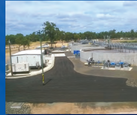
Chinchilla Wastewater Treatment Plant
